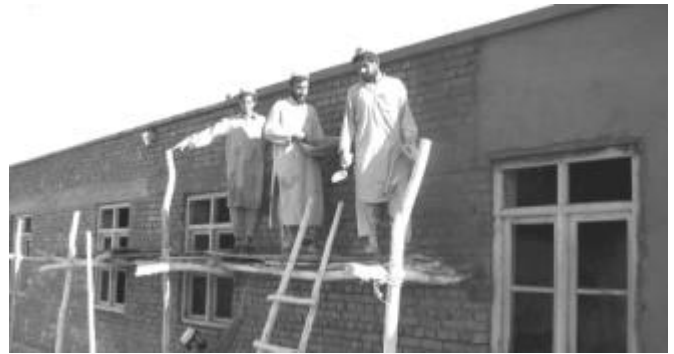
School construction in Afghanistan
